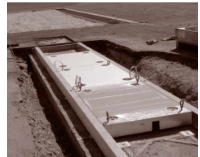
Figure 3. Three force plates installed in the new runway.
